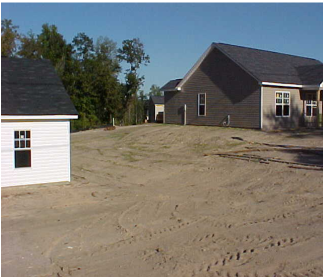
Drainage Around Homes & Yards
