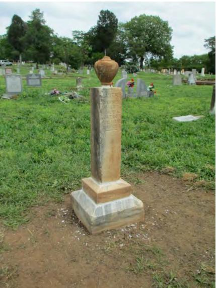
Interned: Merrit Davaul Location: Extra stone, not on list Material: Marble Death Date: 1915 Marker Type: Tablet stone in socket base Condition: Tablet fractured in two pieces and upper portion buried
