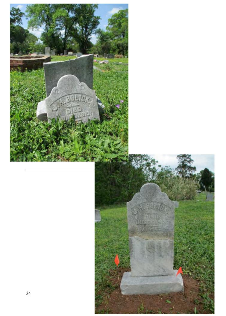
Interned: J.L. Simons, Jr. Location: 437.15 Material: Marble Death Date: 1915 Marker Type: Tablet stone in socket base Condition: Tablet fractured in two pieces
