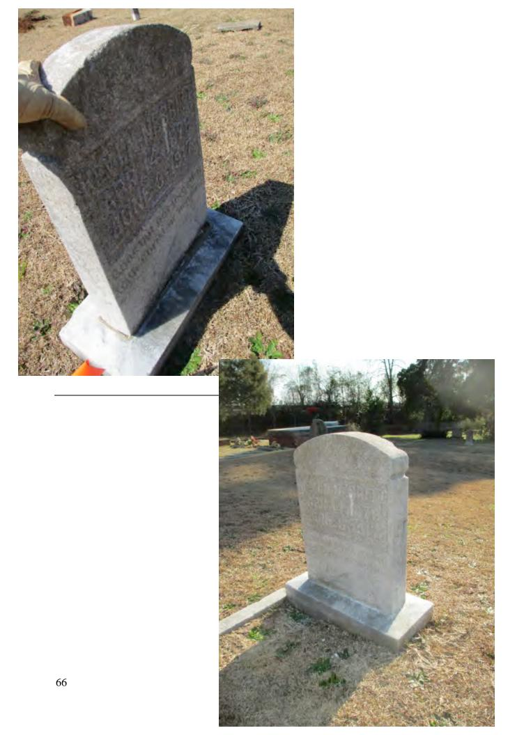
Interned: Robert Richardson Location: 437.16 Material: Marble Death Date: 1898 Marker Type: Tablet stone and socket base Condition: Broken in base, reset in front of base
