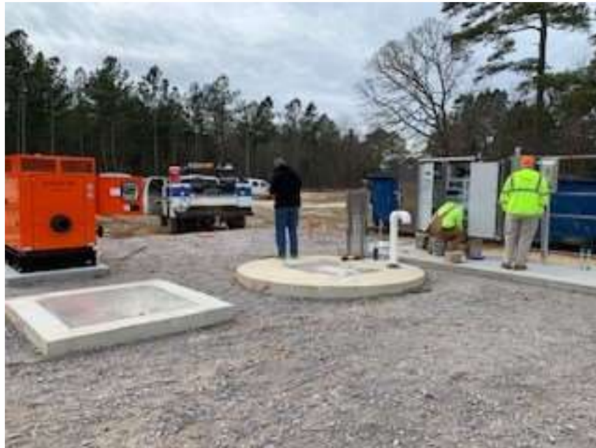
Photo 4: Force main install
