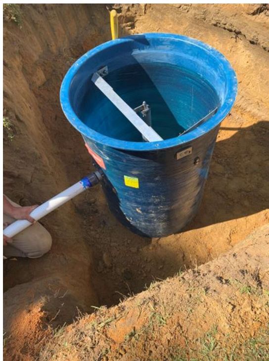
Photo 4: Grinder pump install
