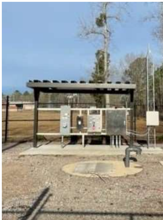
Photo 3: Control panel install
