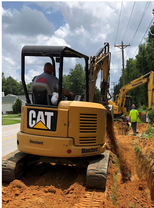
Photo 4: Force main install
