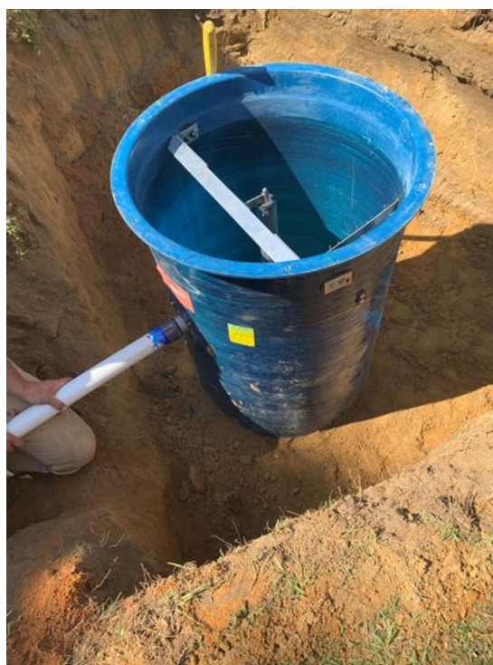
Photo 4: Grinder pump install
