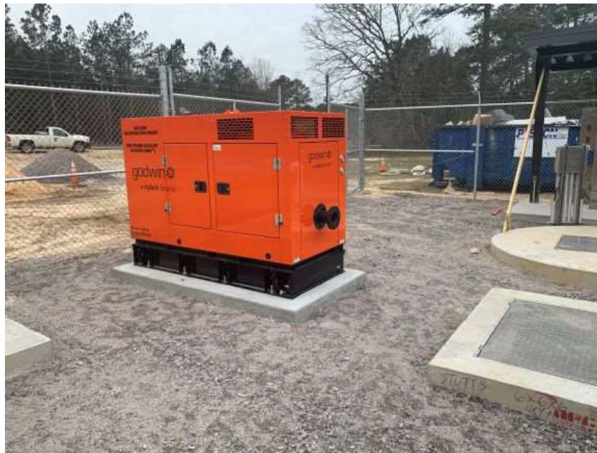
Photo 4: Bypass Pump install
