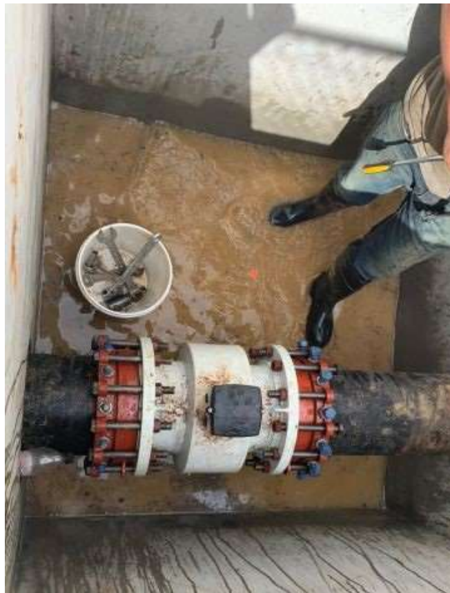
Photo 2: Valve install
