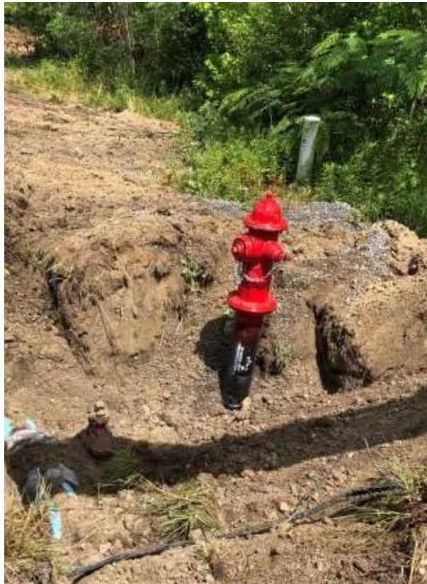
Photo 1: Hydrant install
