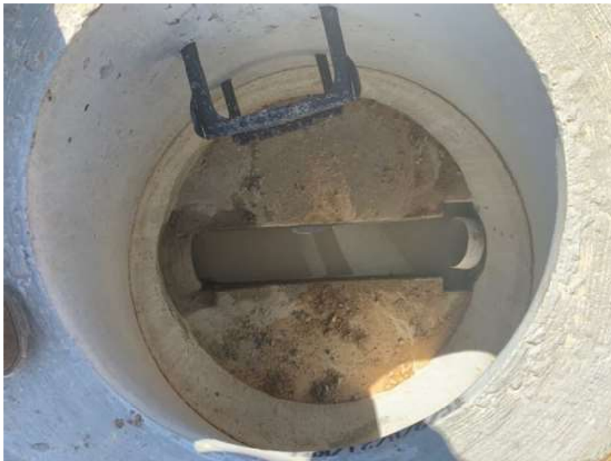
Photo 4: Manhole connection
