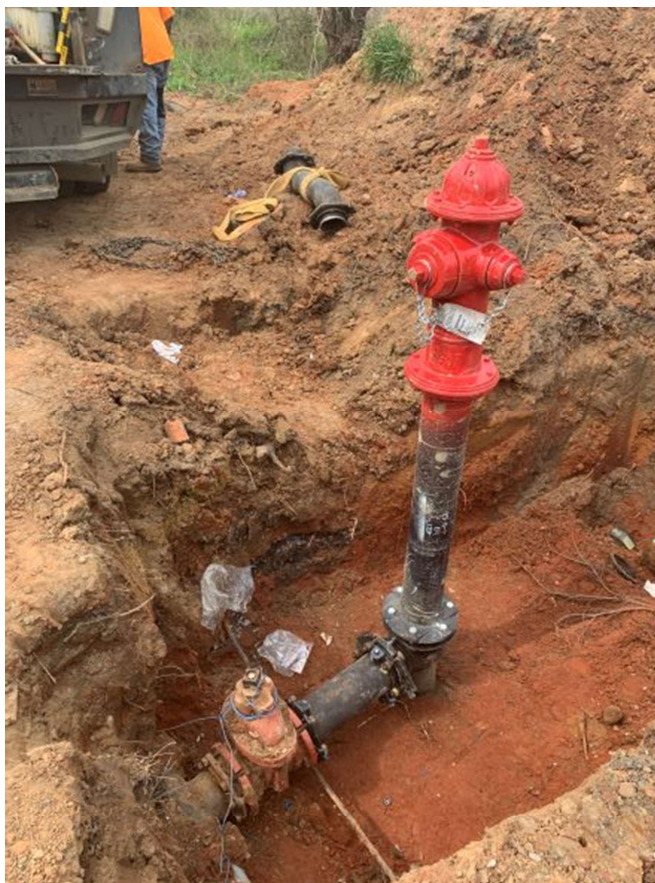
Photo 2: Fire hydrant install
