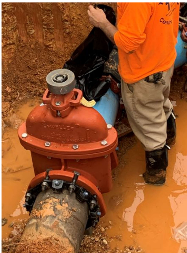
Photo 1: Valve install
