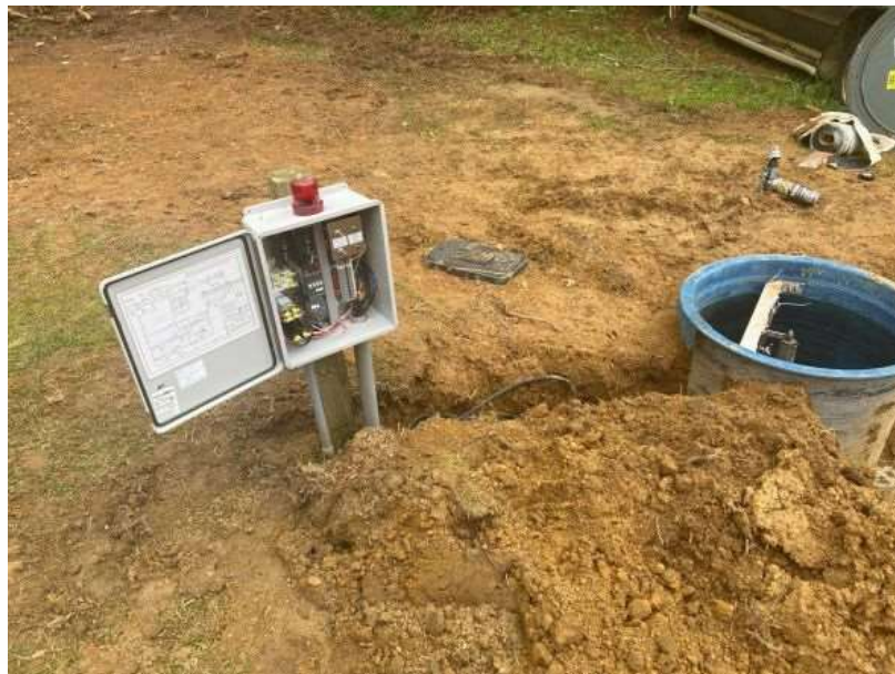
Photo 3: Grinder system install
