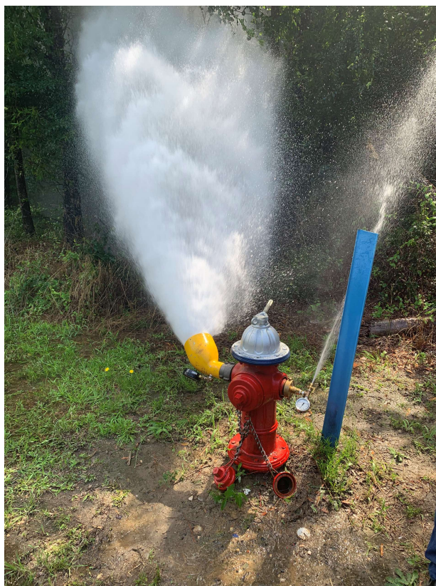
Photo 2: Fire hydrant test
