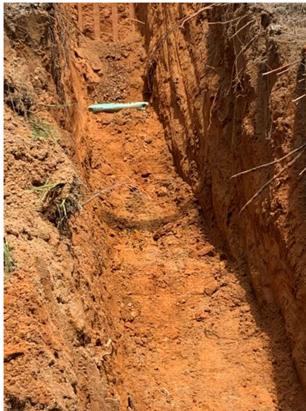
Photo 3: Service connection install
