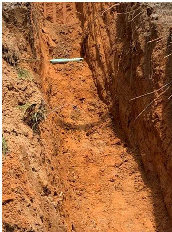
Photo 3: Service connection install
