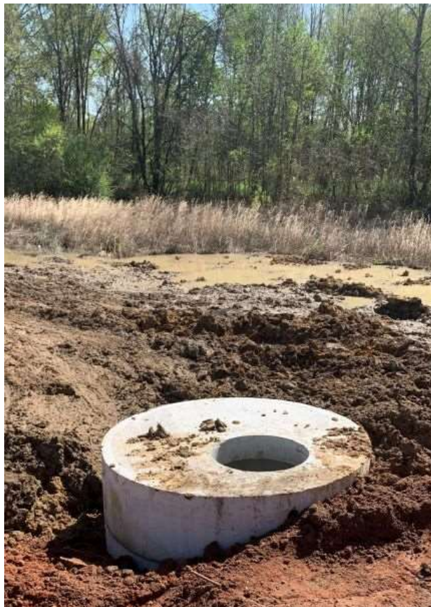
Photo 4: Manhole install
