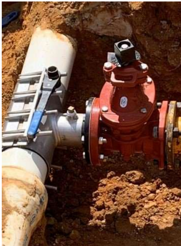
Photo 4: Line Valve installation
