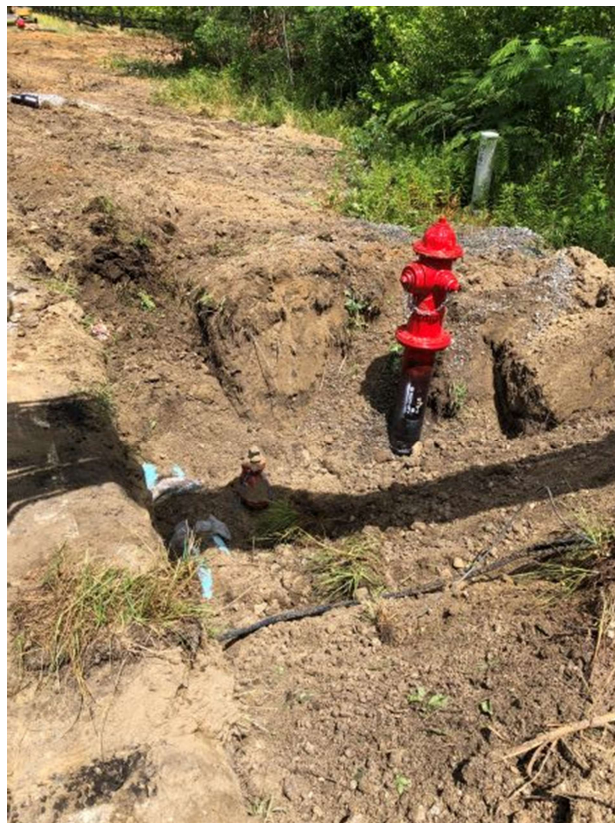
Photo 1: Hydrant install
