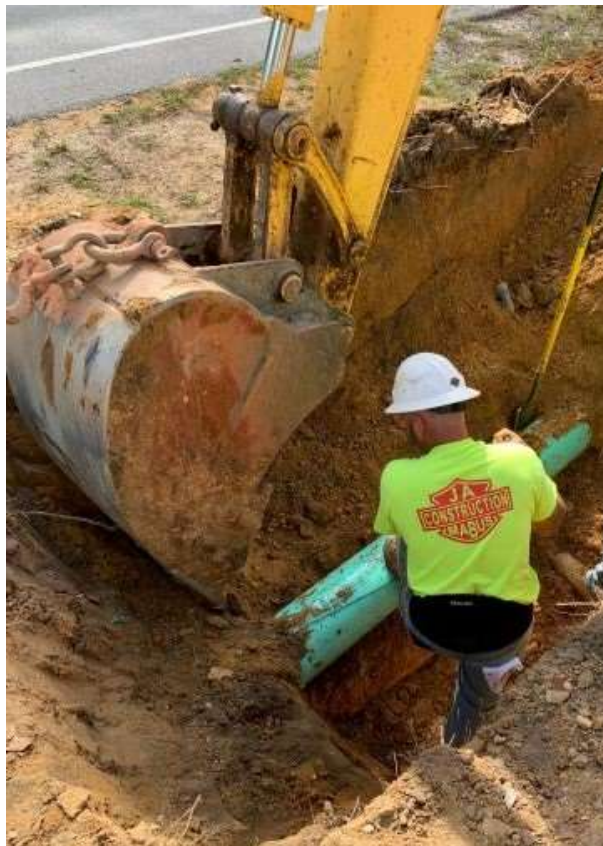
Photo 4: Force main install
