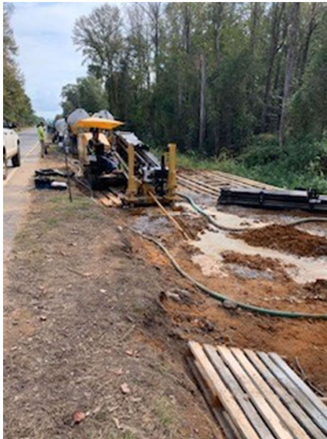
Photo 2: Bore and jack
