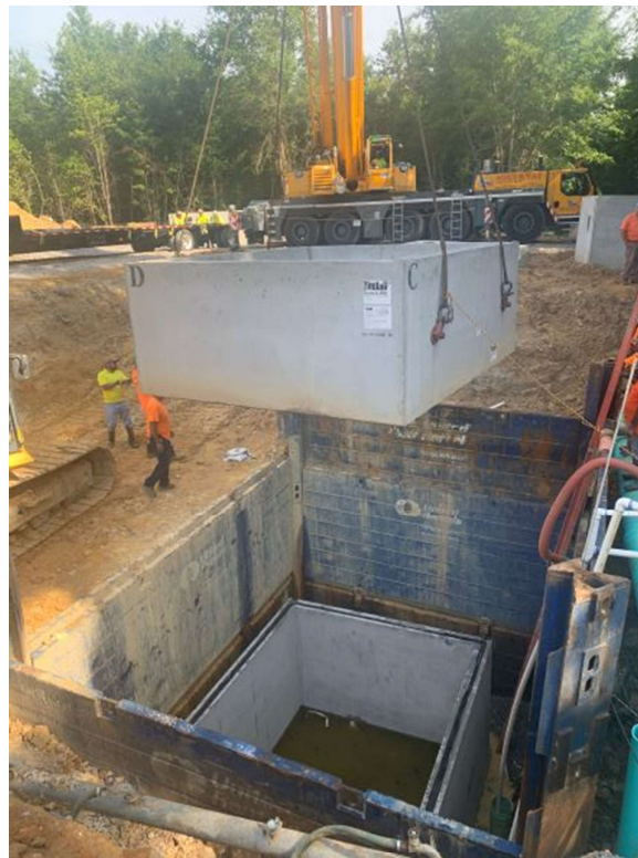
Photo 2: Wet well install
