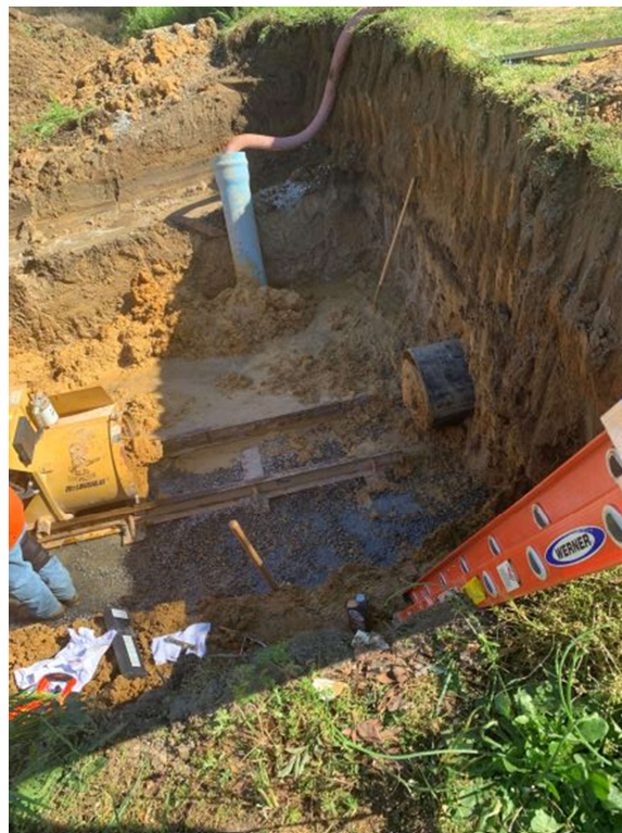
Photo 3: Casing under railroad
