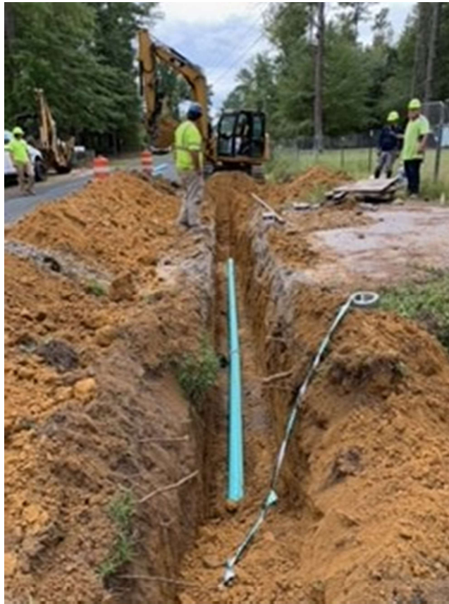
Photo 4: Force main install
