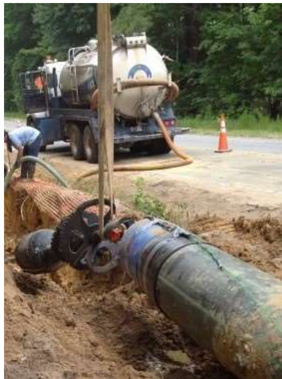
Photo 2: Bore and jack
