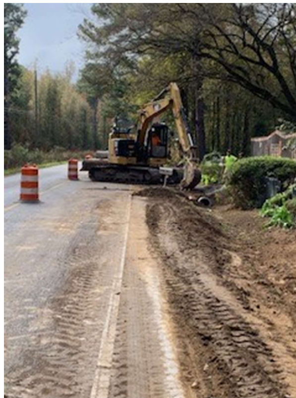
Photo 3: Drain pipe install
