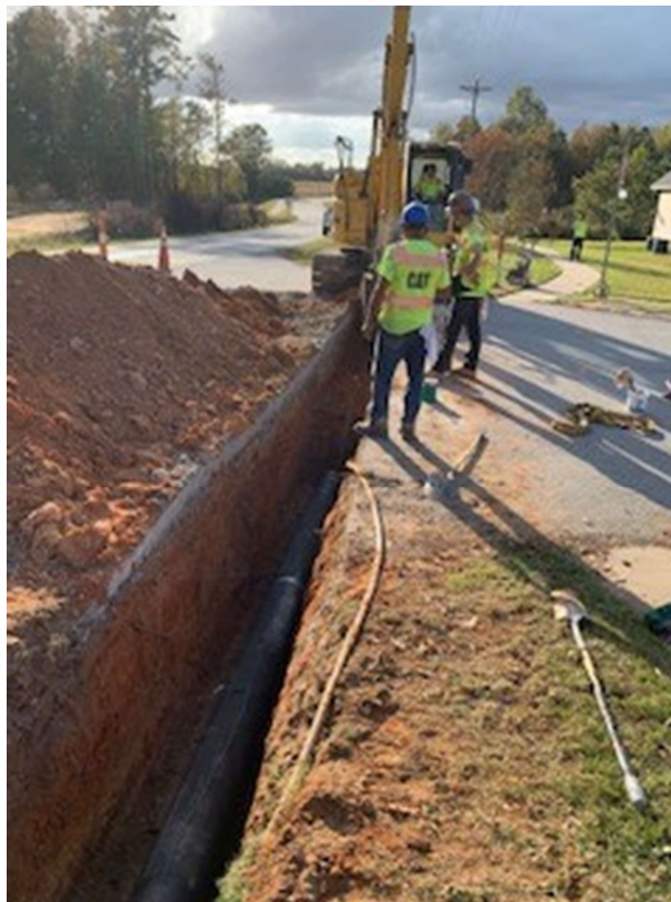
Photo 4: Force main install
