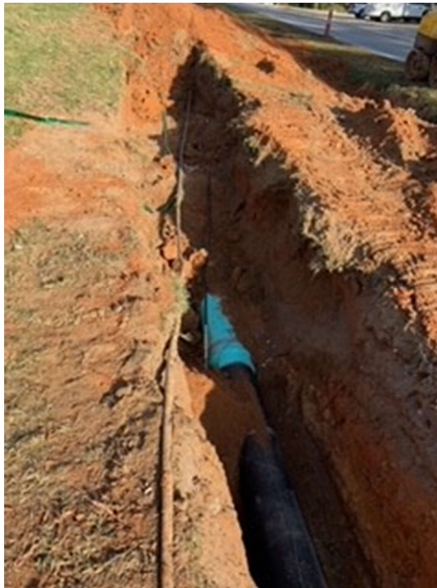
Photo 4: Force main install
