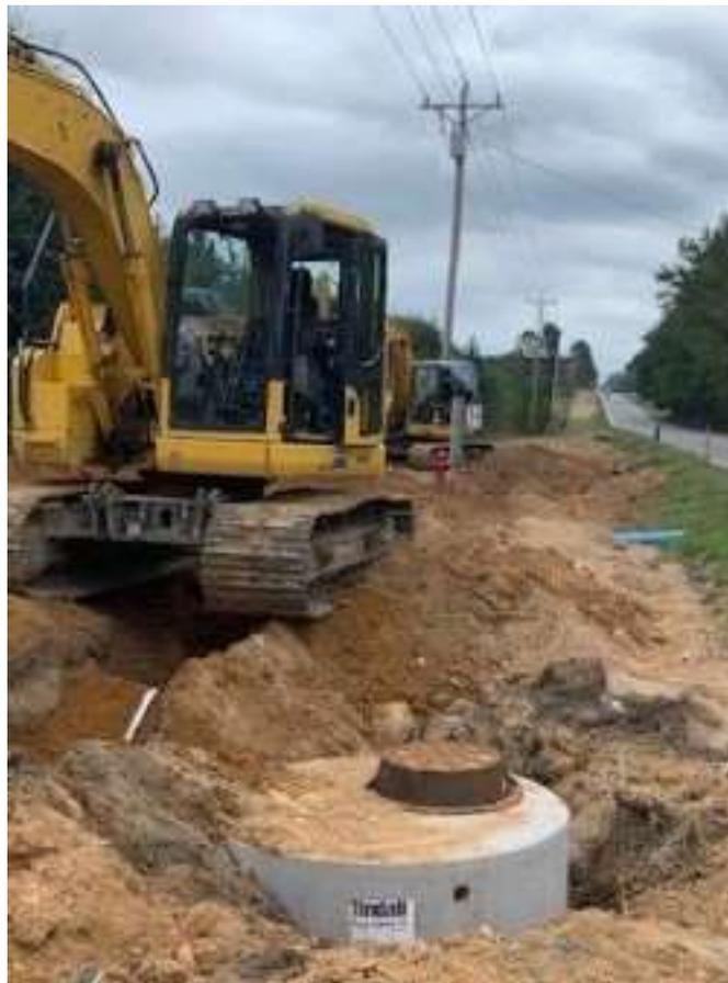
Photo 1: Manhole install
