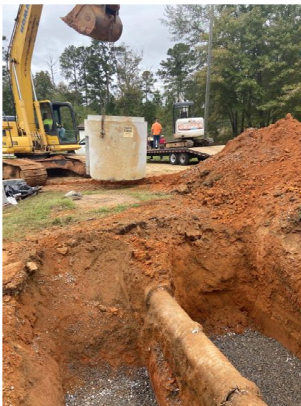
Photo 1: Connector manhole
