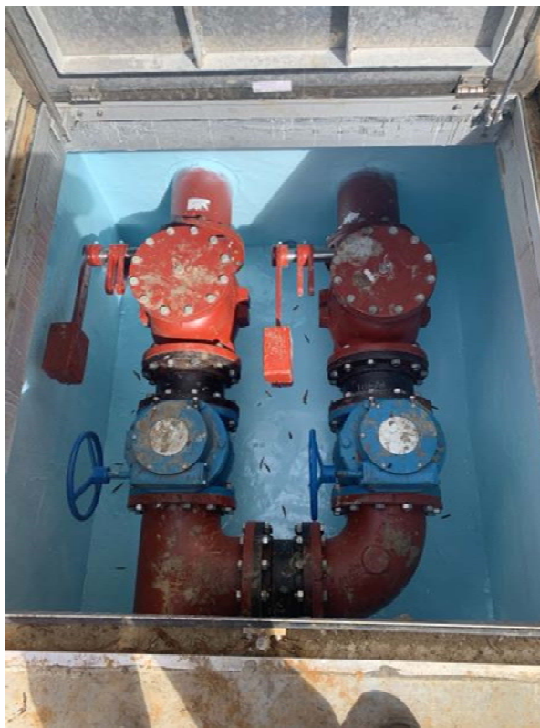
Photo 3: Coating valve pit
