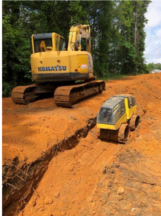
Photo 2: Compaction of trench with wacker
