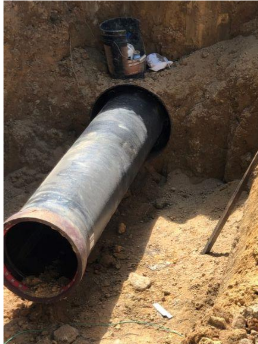
Photo 1: Bore under Horrell Hill Road
