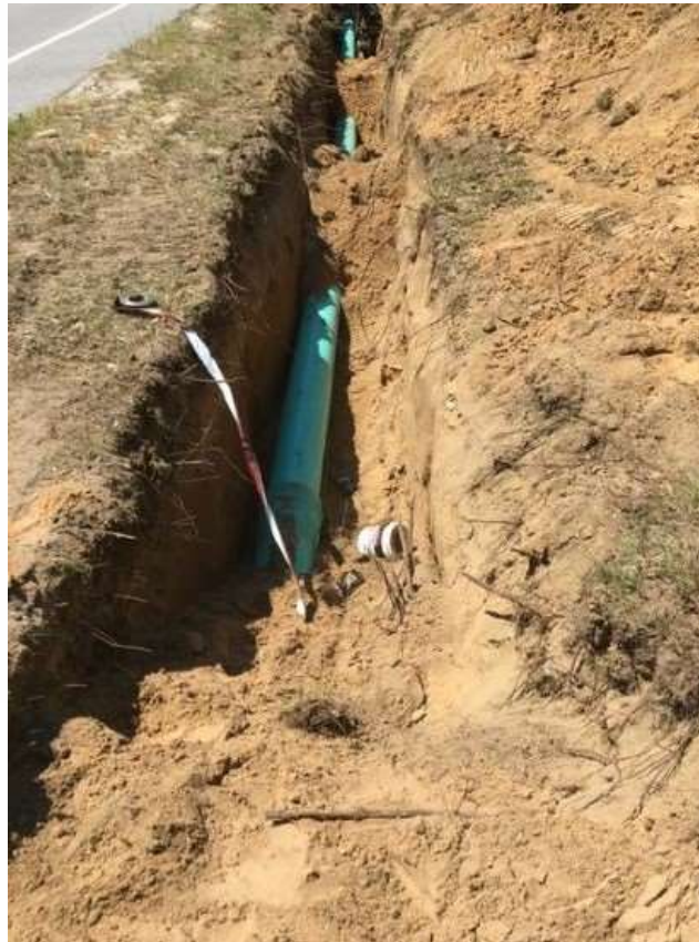
Photo 4: Force main install
