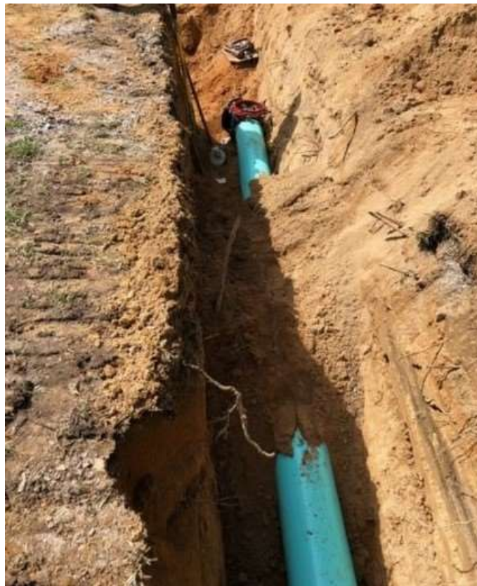
Photo 4: Force main install
